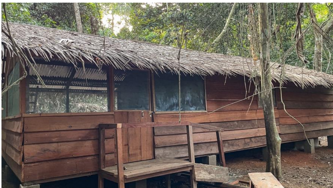
A new house at Dzanga bai for the research team ©Nuria Ortega
