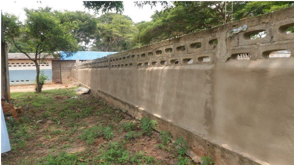
The hospital is now better protected © Luis Arranz
