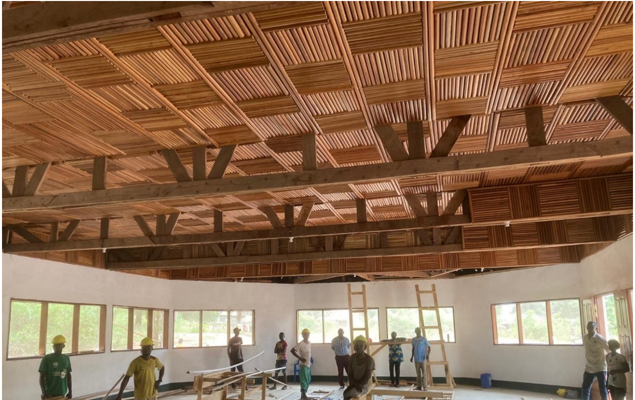
New ceiling in the PAPA hall © Luis Arranz
